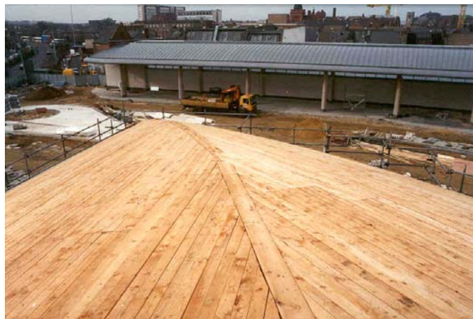
Figure 4 – Bus Station under construction in Sunderland
